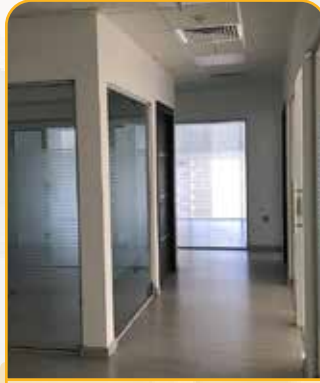
Low & High Partitioning Works
