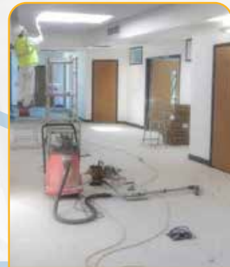
Post Construction Cleaning
