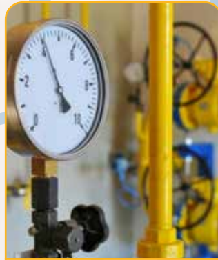
Building Plumbing Work
